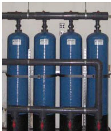
The full weight of the piping and valves must be supported by unistrut, pipe hangers or other means. The tank connections can not support the weight of the piping. This photo from a multi-tank system installation shows properly supported piping.
